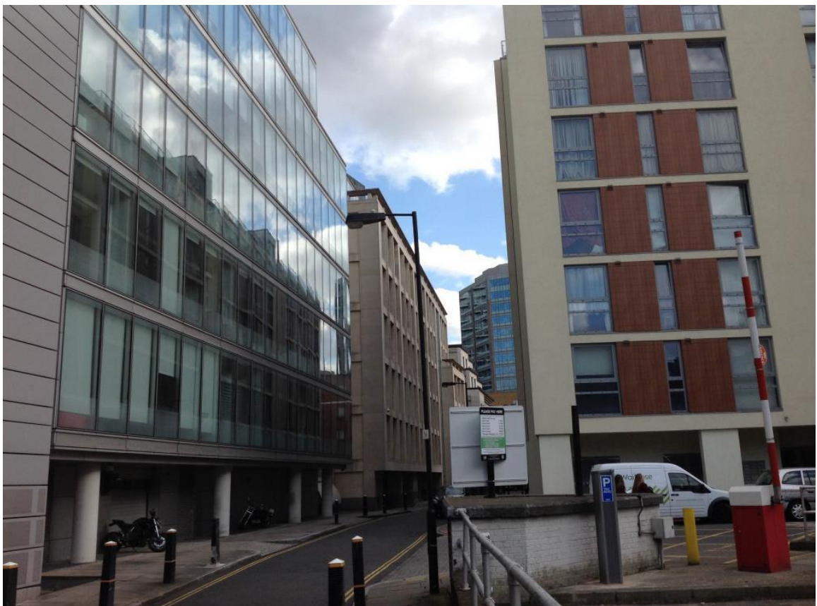
View of adjoining buildings facing the application site with Lamb's Passage to the left and Sutton Way to right.
